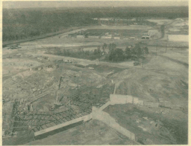
Land Pavilion first steel.
